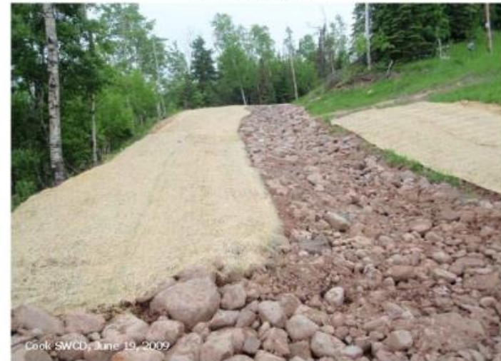
Trailside Ditch Stabilization, Riprap and Reseeding - After Ullr Mountain
